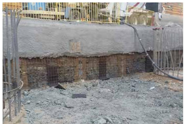
*Drilled piers on either side of the excavated bedrock with the first phase of shotcrete applied.*
