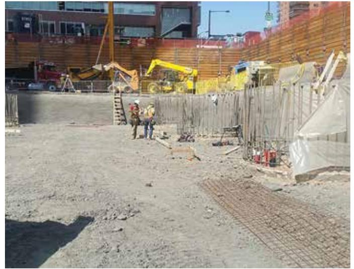
*Team members prepare to form the tie beam system that will support the foundation of 1144 Fifteenth Street. The bedrock is covered with an earth retention system and shotcrete; drilled piers line the top and right.*
