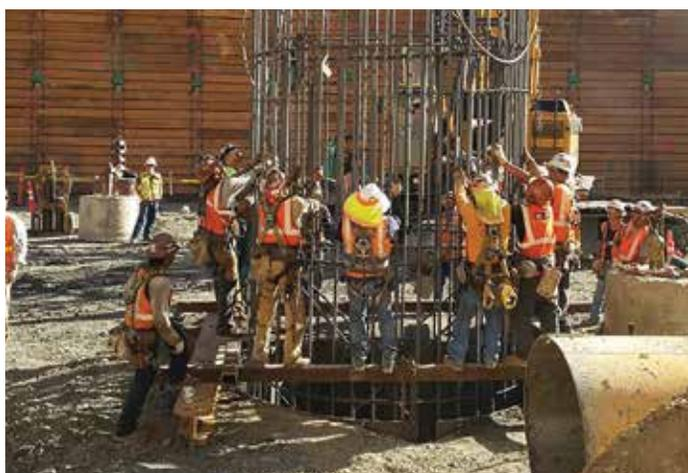
*Workers splice together two sections of reinforcing steel that form drilled piers used in the foundation for 1144 Fifteenth Street.*
