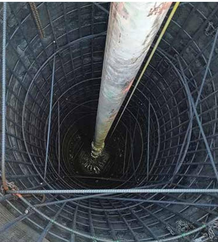
*A downhole view of the reinforcing cage and concrete placement for a drilled pier used in the foundation for 1144 Fifteenth Street.*
