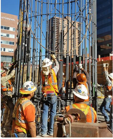
Workers connect sections of the reinforcement cages to be set in the 100-foot deep pier footings.
