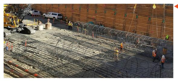
Reinforcement cages are ready to be lowered into the drilled pier holes.
