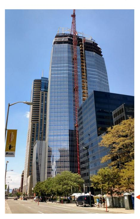
Construction of Denver's fourth tallest building calls for innovative solution to compensate for soft sedimentary bedrock.
