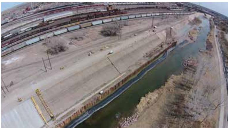
**Fig. 2:** A hydrologic study showed that the Pueblo levee could be lowered. The original height and narrow top of the levee can be seen in the background (upstream). The toe of the downstream portion of the levee was found to be below the river level, so sheet piling was used to provide access for construction of the new concrete facing
