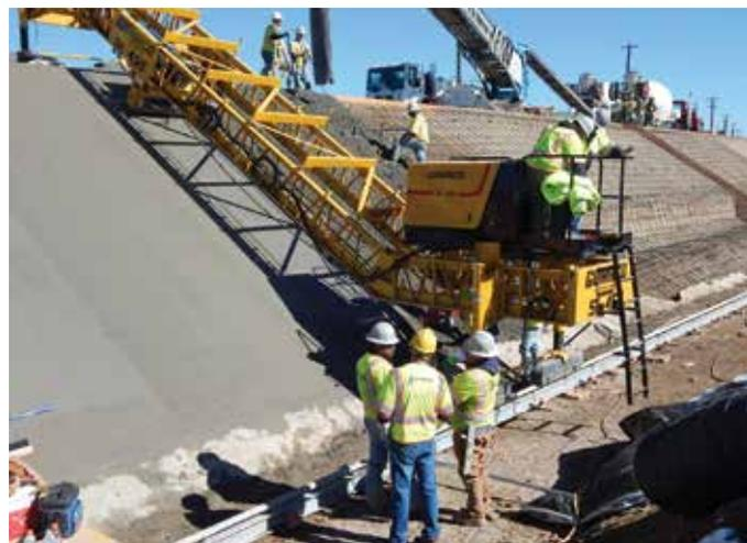
**Fig. 3:** The lowered levee provided a wide access way for concrete delivery. Concrete trucks were routed up a temporary access embankment and delivered concrete to a conveyor that placed the zero-slump concrete mixture ahead of the canal paver
