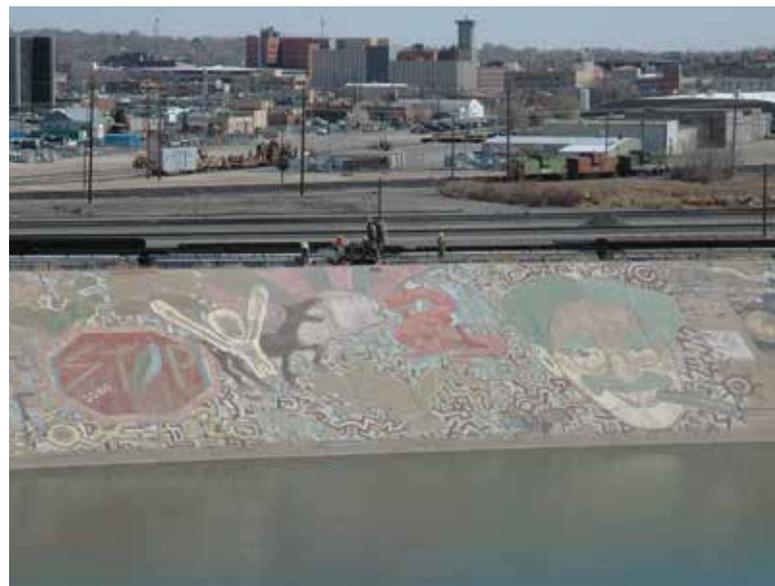
Fig. 1: The river side of the levee in Pueblo, CO, included a large mural produced by multiple artists. The levee was evaluated with the aid of borings taken with a narrow-track drilling rig (center)
