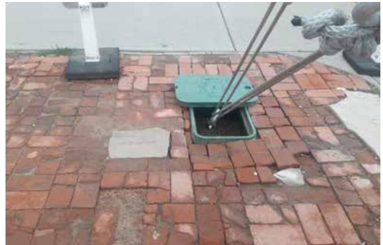
The helical pile system is hidden with a manhole cover or sprinkler valve box when not being used.
