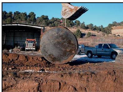
CTL coordinated the removal and disposal of an underground storage tank (UST). Services that were provided include soil sampling, removal and disposal of the tank contents, and the facilitation of regulatory closure with the State of Colorado.
